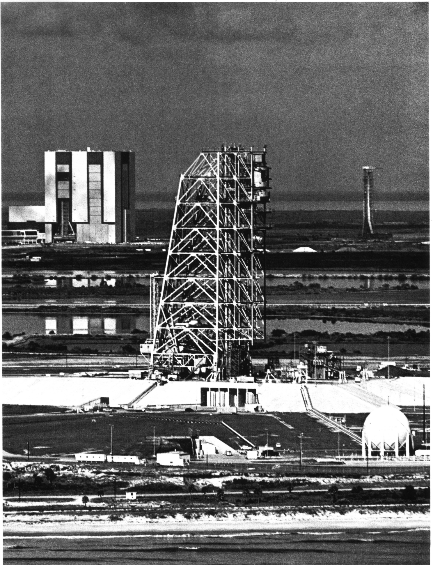
Complex 39, Kennedy Space Center, Fla., is jump-off for first flight of Apollo 4 and for future moon missions. Fully assembled, checked-out space vehicle moves on crawler from Vehicle Assembly Bldg., background, along custom-built road 3.5 miles to launch site.
